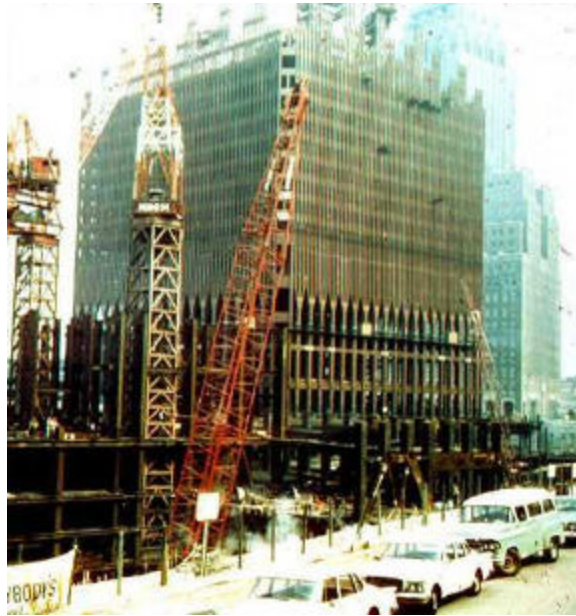
Figure 6: Towers under construction (www)
