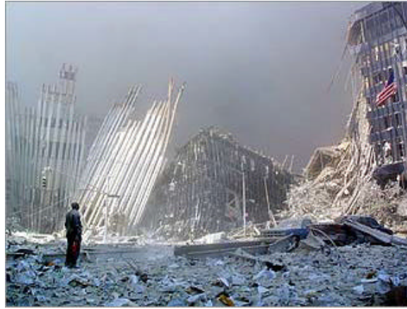
Figure 4: Collapsed tower with perimeter columns still linked at the bottom floors (www)
