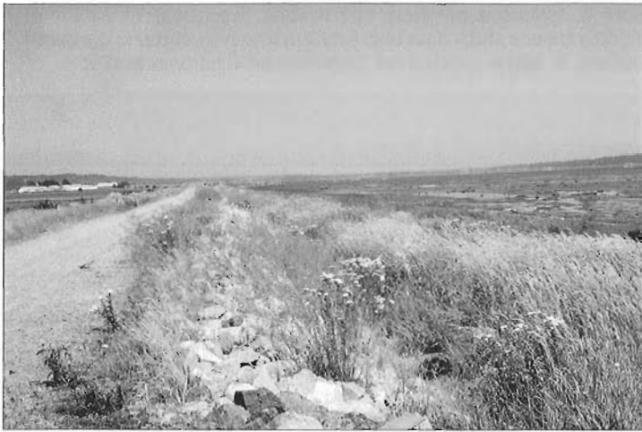
Figure 8. Physical constraint to landward saltmarsh migration under rising sea levels: the sea dykes of Boundary Bay. Photograph by M. Dunn, Canadian Wildlife Service.
