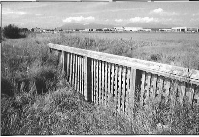
Figure 7. Debris screen at channel opening of constructed marsh, Middle Arm, downstream of No. 2 Road Bridge. Photo by M. Adams. GSC 2003-499
