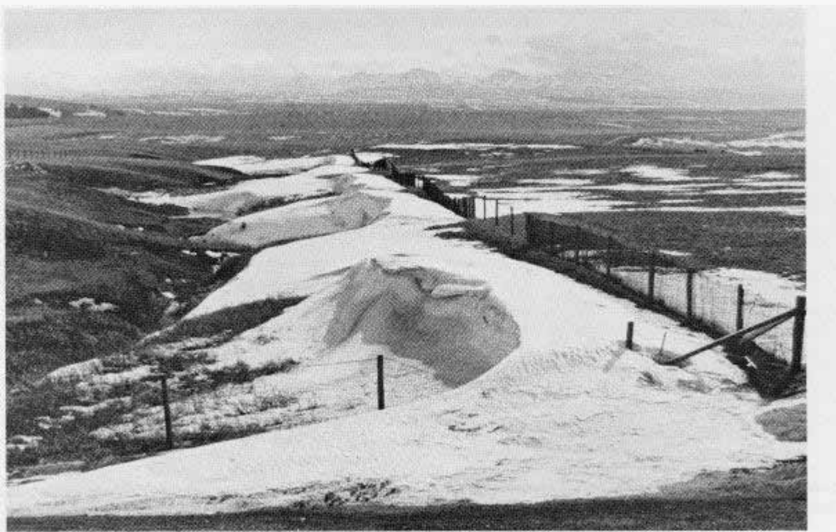
Snow fences as part of the mitigation program (Photo Alberta Public Works Supply and Services)
