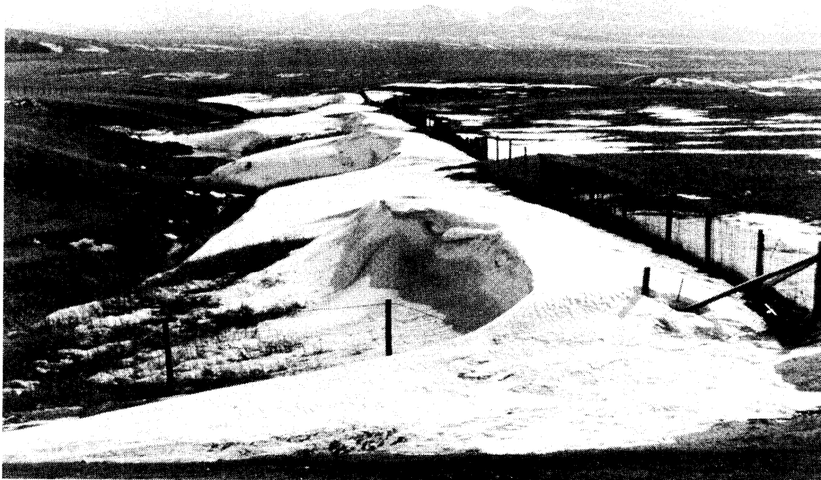
Snow fences as part of the mitigation program (Photo Alberta Public Works Supply and Services)
