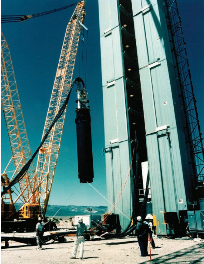
Workers prepare for the last U.S. nuclear test, "Divider," a Los Alamos–designed shot that took place on September 23, 1992. Here, the Divider device is shown before being lowered into its test shaft. When the device was in place, the shaft was filled with layers of magnetite, sand, concrete, and epoxy to contain the bomb debris underground. (Photo: Los Alamos)
