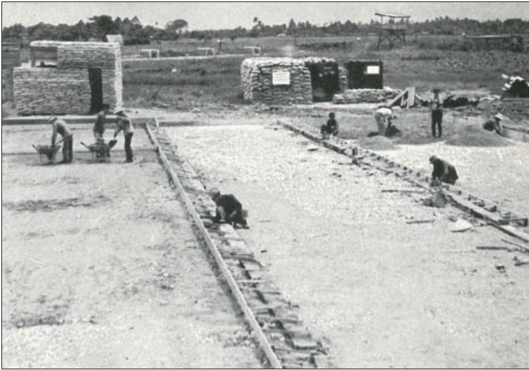
(Left) R&U Construction Crew Laying Warehouse Foundation at Vinh Long in the Mekong Delta—Guard Tower and Bunkers have been Built for Security in this Remote, Hostile Area. (Right) Vietnamese Women Being Trained as Welders—the Instructor for the R&U Contractor and a Vietnamese Interpreter-Assistant are Shown at the Left.
