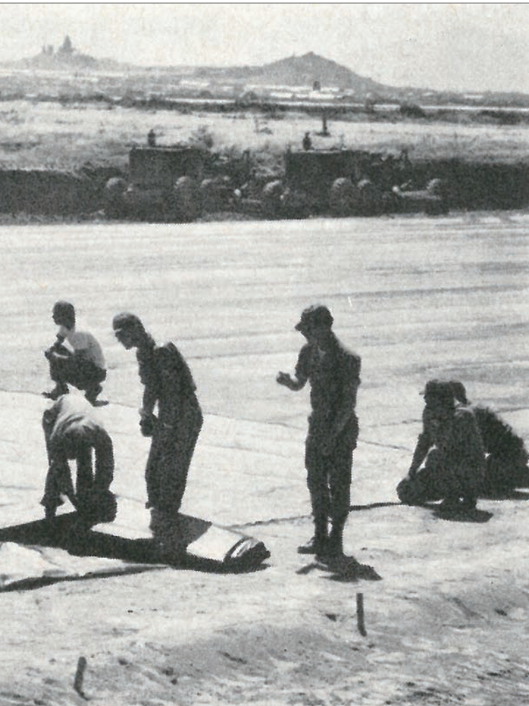
(Top) Preparations of the Site for Runway Concrete Anchor (Left) Nylon Membrane Being Placed on Runway Prior to Laying Mat
