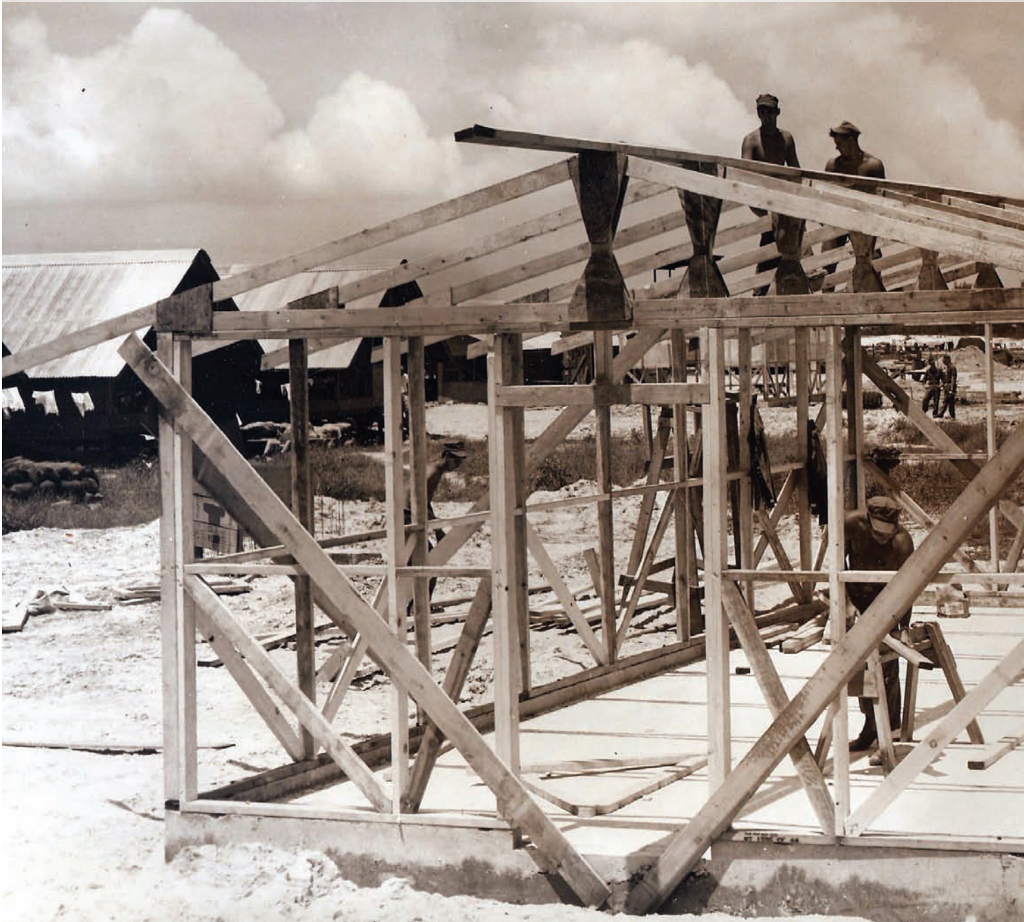
Seabees with Naval Mobile Construction Battalion 7 build a shower facility in Phu Bai, Republic of Vietnam, 1966. U.S. NAVY PHOTOS
