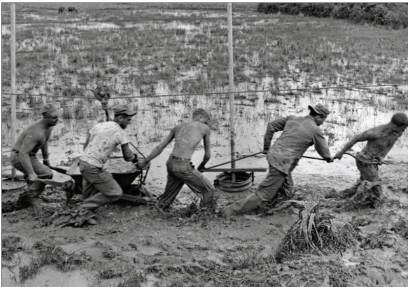
Personnel from Delta Company, Naval Mobile Construction Battalion 128, plow through a rice paddy as they set fence posts at Ammunition Supply Point #1, Da Nang, Vietnam. Delta Company provided perimeter security in the form of a 6-mi chain link fence that was put up over terrain that varied from rice paddies to the sheer slope of a rocky hillside.
