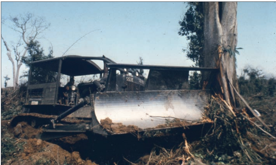
This Rome plow unit, one of the first six to be used in Vietnam, clears vegetation from the maintenance and supply area in the Long Binh complex, November 1966.
