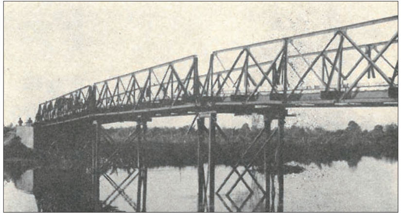
Steel Bridge in South Vietnam.
