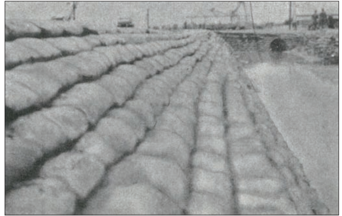
Figure 2. Sandbagging with Soil Cement and Sand Mixture
