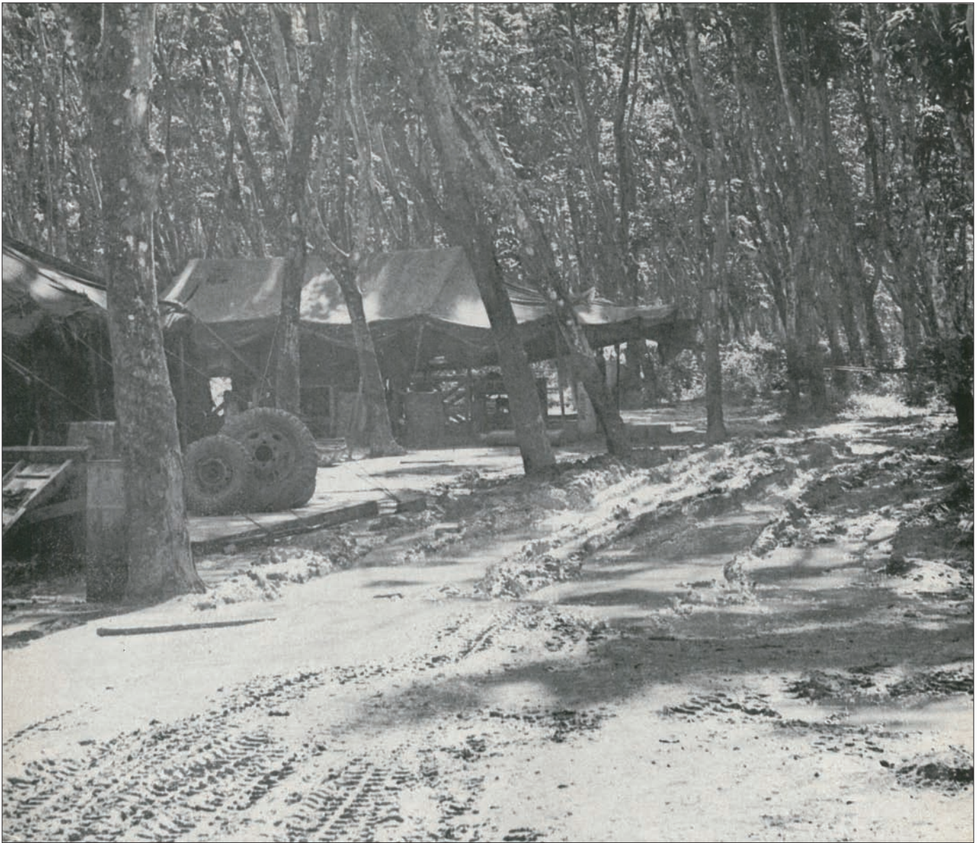
This was the beginning of the R&U installation at Lai Khe, about 40 miles from Saigon. Tents were—and in places still are—the R&U contractor's only facilities at many installations in Vietnam.
