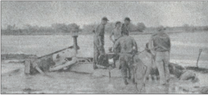
Figure 5. Tractor Sinking in the Fill
