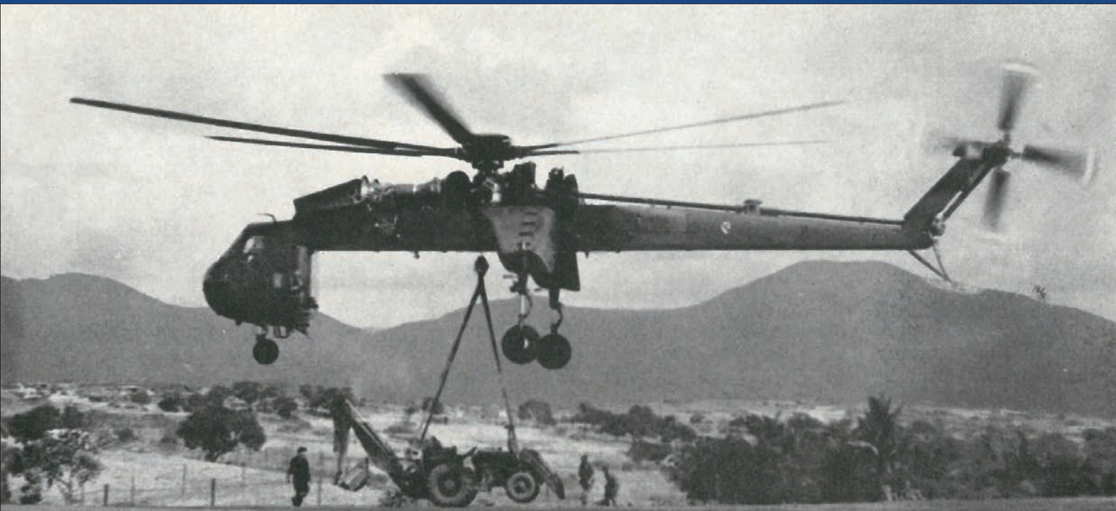
CH-54 "Flying Crane" Lifting Construction Equipment for the Dusseau Airfield
