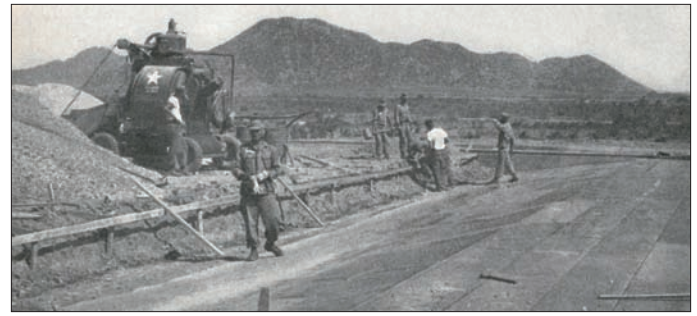
(Top) Preparations of the Site for Runway Concrete Anchor (Left) Nylon Membrane Being Placed on Runway Prior to Laying Mat
