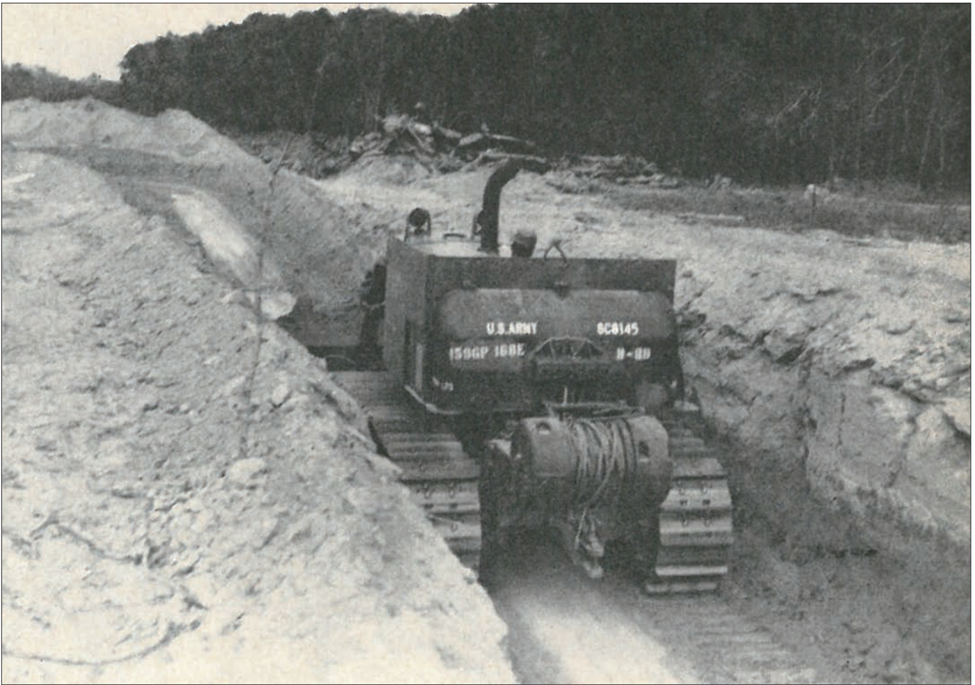
Earthwork on an Airfield at Lai Khe
