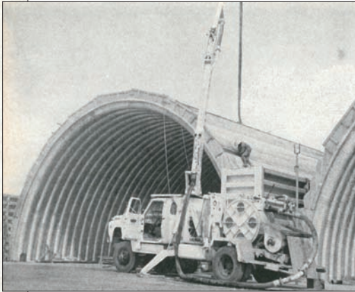
(Top) Figure 1. Placing Concrete from Pump Truck with Boom and Tube (Left) Figure 2. Completed Shelter Housing F-100 Jet Aircraft (Jet Blast Deflector in Rear)
