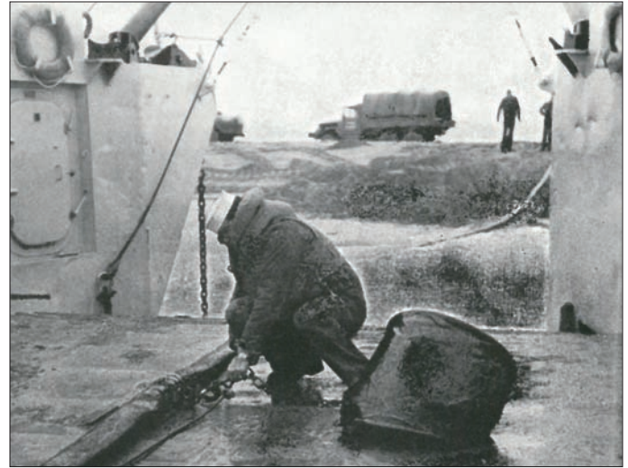
(Left) Ready to Attach Hose to Tension Relief Cable as Both are Wound Off the Reels in Launching (Right) Attaching a Floater Buoy to Hose at 50-foot Interval as the Hose and Cable Are Payed Out
