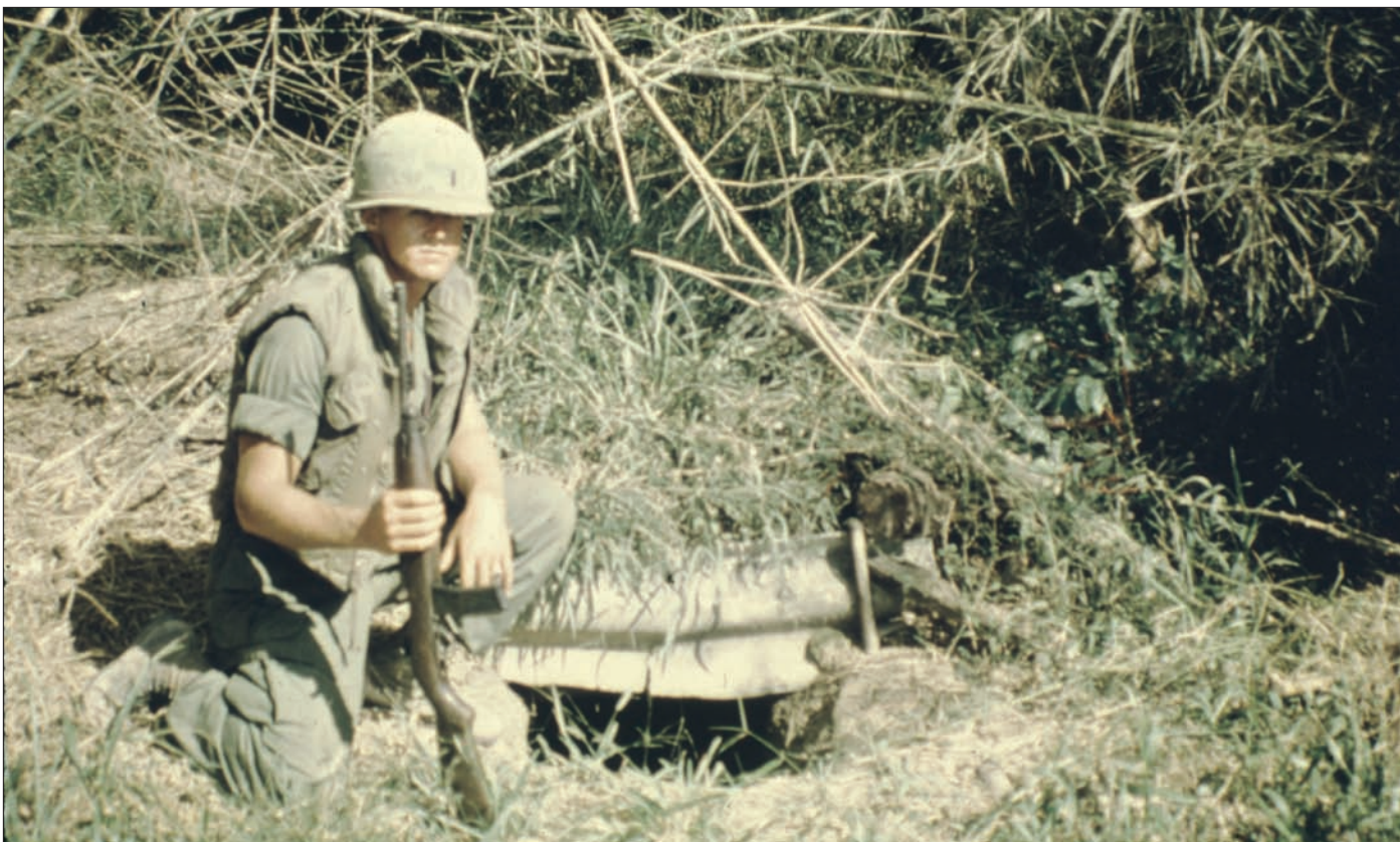
1st Lt. William Gang of the 168th Engineer Battalion's Land Clearing Team, "The Jungle Eaters," kneels next to an opening of a tunnel complex discovered in the Iron Triangle during Operation ATLANTA, December 1967.
