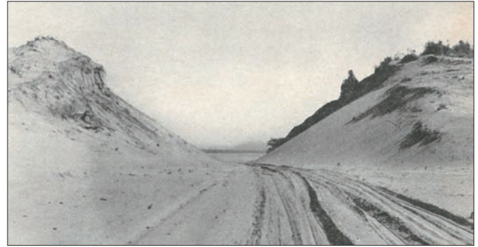
Temporary Road as First Constructed
